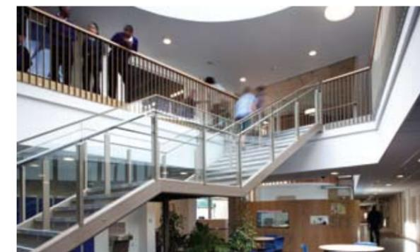
concrete soffits and walls reduce the need for expensive and maintenance-heavy finishes and provide thermal mass to reduce energy needs. The new building generates 20 per cent of its energy from on-site renewable energy installations.
